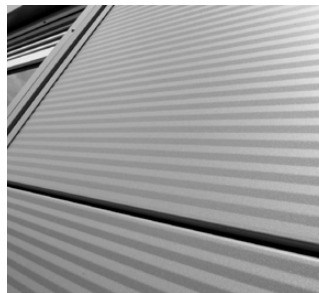
Horizontal Micro-rib Composite Cladding.
