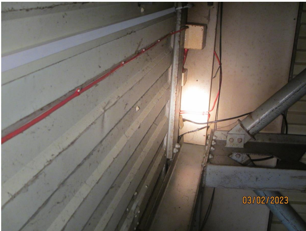
Photo 12. Sheltered features within Building 1 were inspected thoroughly and no evidence of roosting activity was identified.
