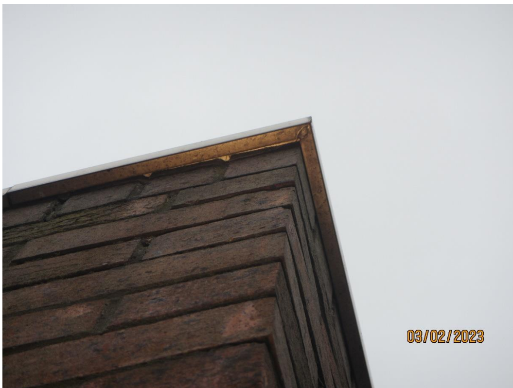
Photo 14. The wall plate of Building 2 is capped and tightly sealed to the brickwork.
