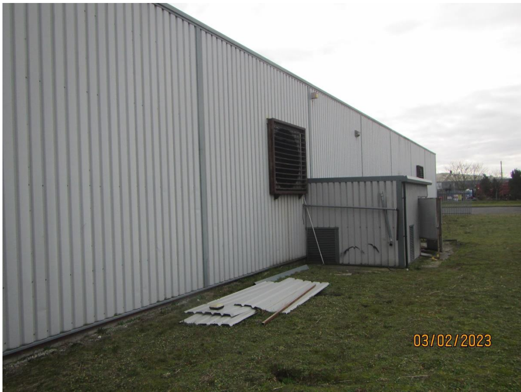
Photo 10. Western aspect of Building 1 with corrugated materials visible that were inspected for evidence of reptiles or amphibians.
