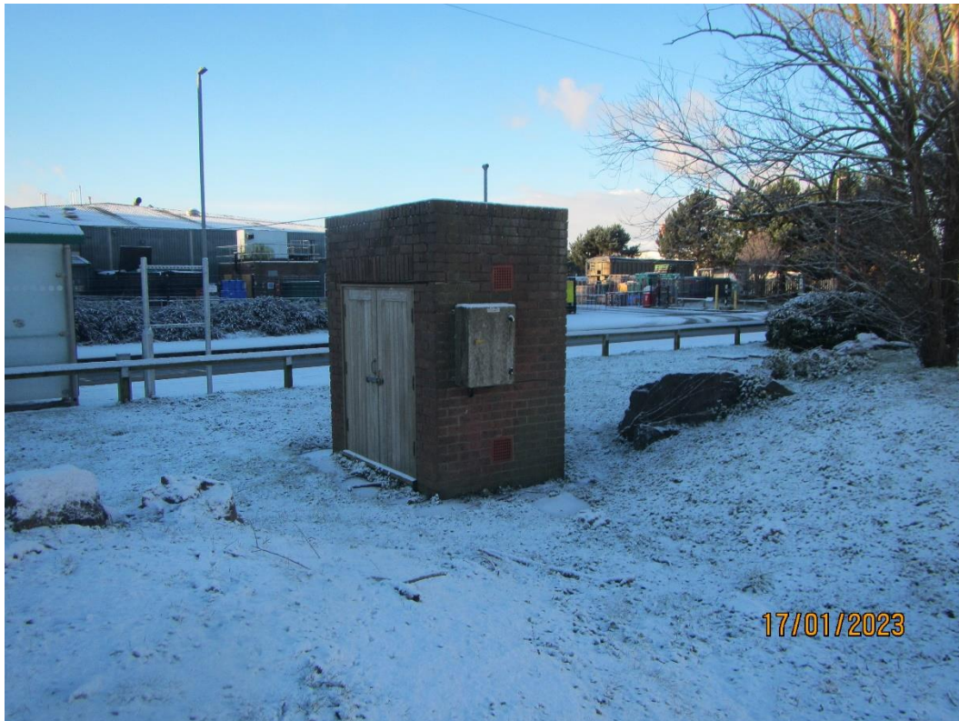
Photo 15. Northern aspect of Building 3, which is another redbrick substation.
