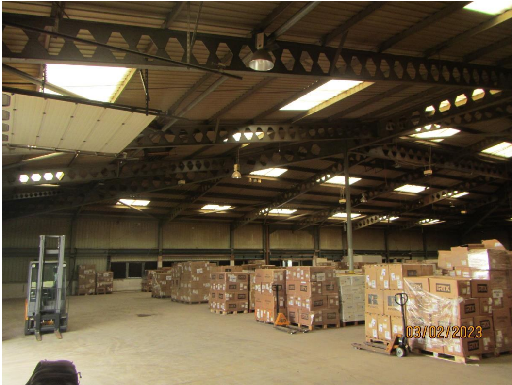
Photo 11. Interior of Building 1 showing the large levels of natural light.
