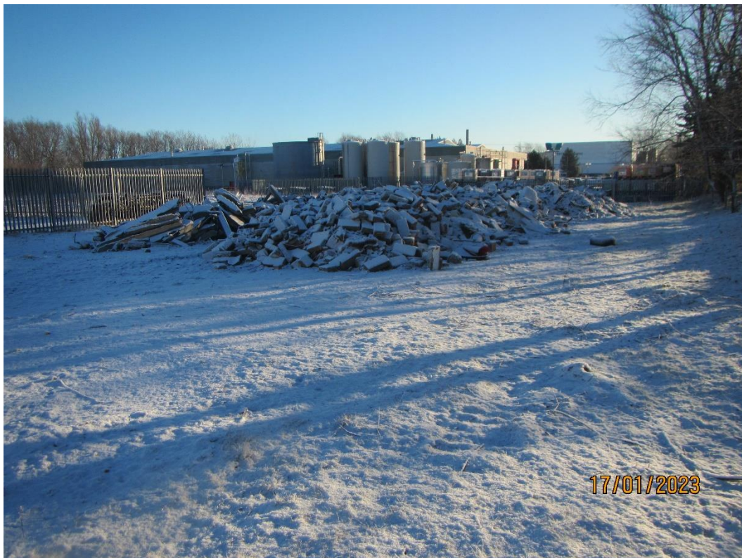
Photo 18. Concrete blocks and other debris at Target Note 5.
