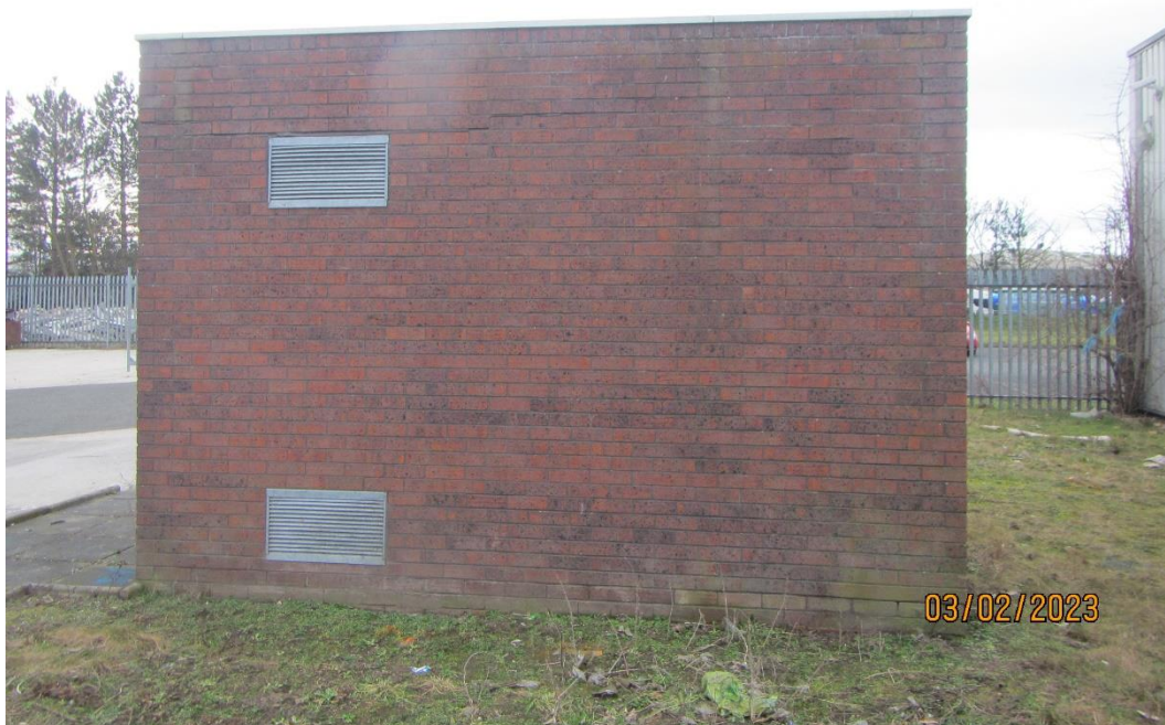
Photo 13. Northern aspect of Building 2, which is a red brick substation.
